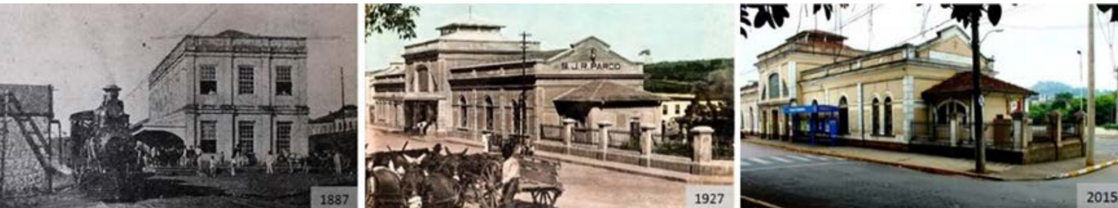
Figure 5. São José do Rio Pardo Central Station.
